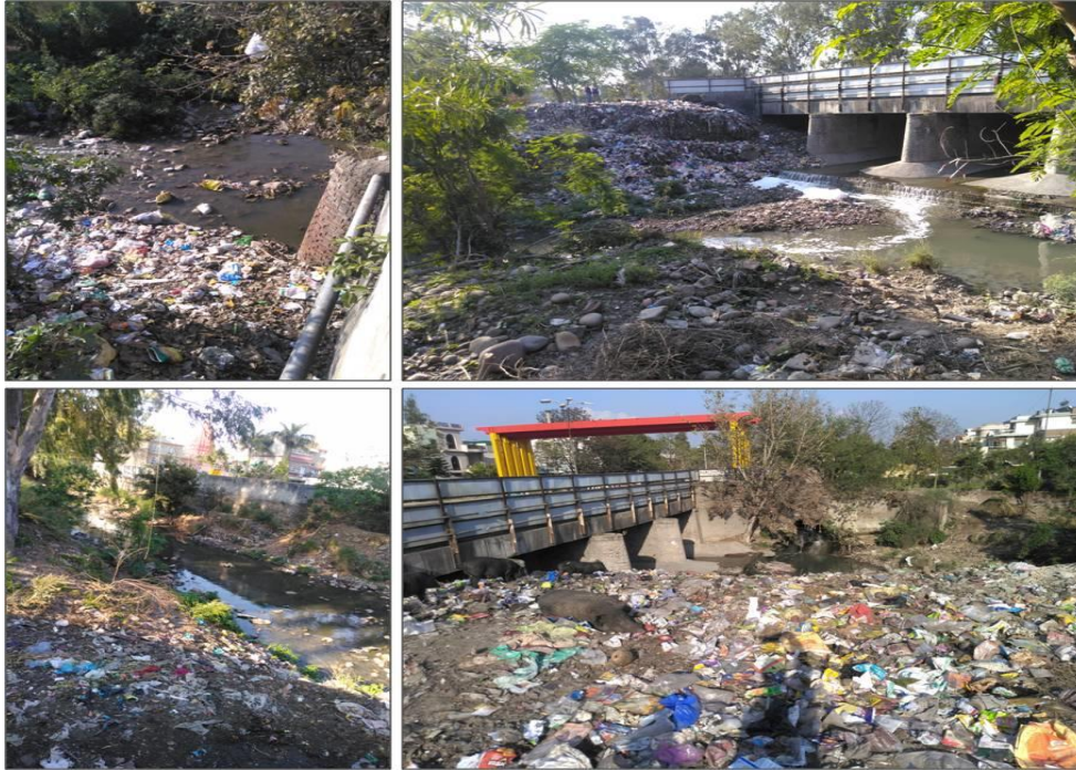
Figure-8 Solid Waste into drain at bridge near Sector-18, Panchkula.
